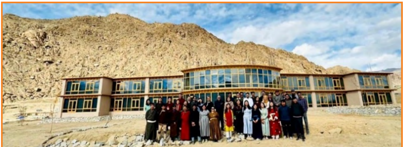
Administrative block of the School of Sustainable Habitats in Himalayan Institute of Alternative Learning (HIAL), Ladakh
